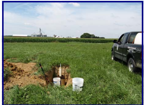
Soil drainage testing
