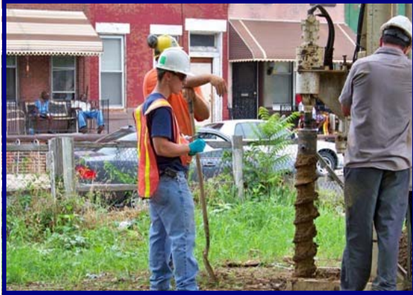
Testing subsurface conditions prior to redevelopment
