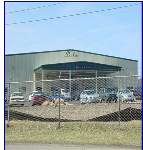
After remediation activities
